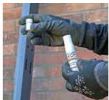
1. Remove the small powder coating pot from the top of the touch up stick.
