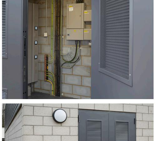
door panels that allow for up to 50% airflow. In this case, the panels were fitted to Steeldor double and single doors without effecting the levels of performance or high standards of quality.
